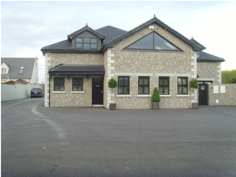
Figure 1 – Building where heat pump is installed
